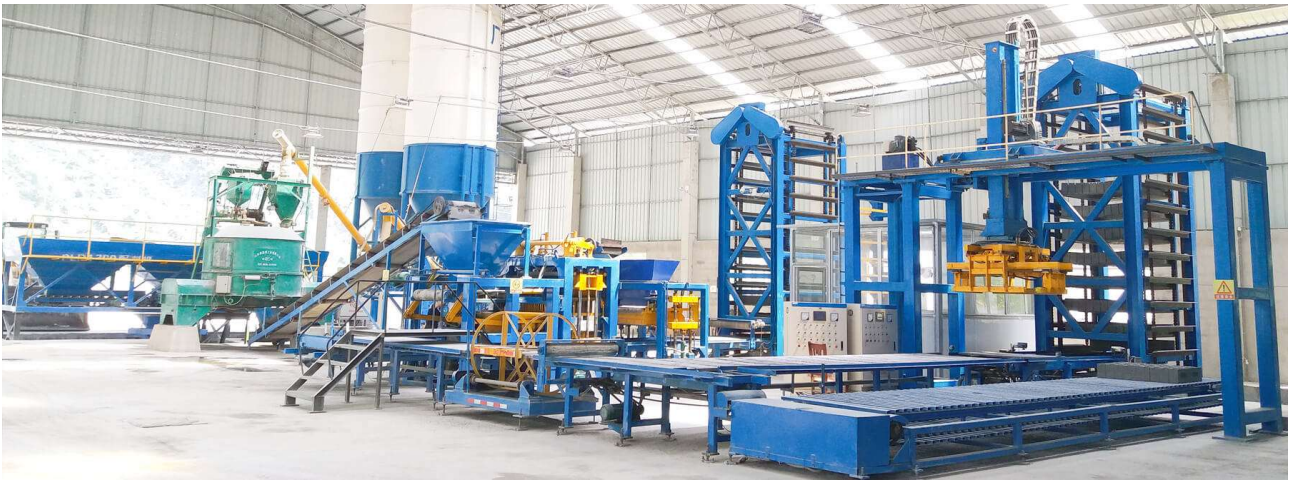
Full automatic concrete block manufacturing plant
